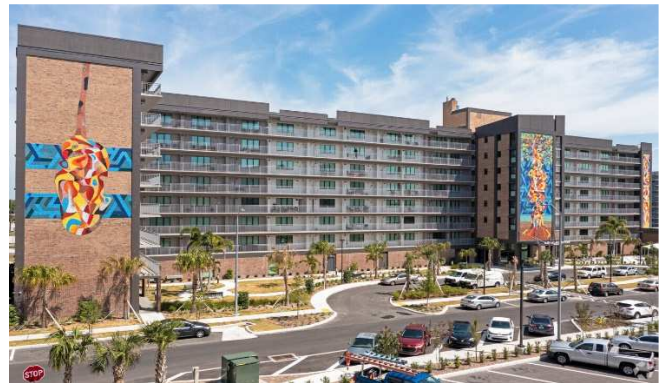
THA's Newly renovated Mary Bethune Highrise
