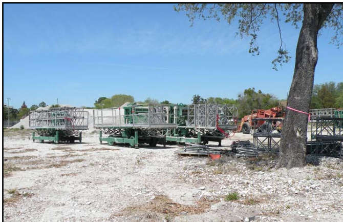
Contractor staging on site
